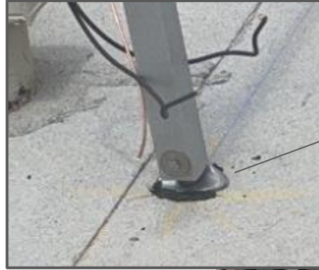
Racking with Weather proof Sealant
